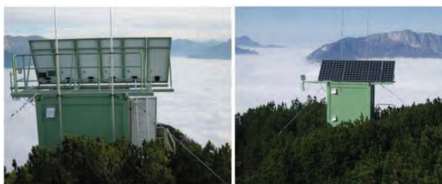
Figure 3: Additional autonomous GATE transmit stations GTS 7 & 8
